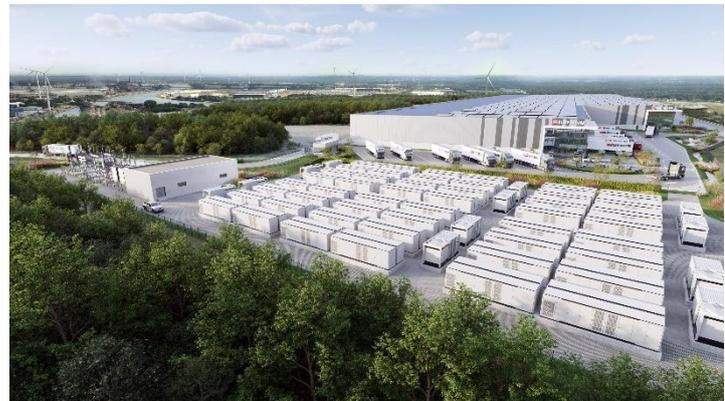
The battery park has a total capacity of 60 MW (being the maximum power the system can absorb or deliver at any given moment), and up to 240 MWh energy storage capacity. Therefore, at full output, the battery can operate for four hours.
