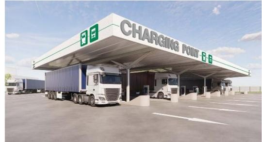
In Bleiswijk, the Netherlands, WDP is developing a next-generation electric truck charging hub in partnership with Einride. The site, which will be operated by Einride upon completion end-2026, will offer six high-power charging points with 600 kW of simultaneous charging capacity.
