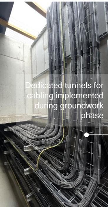
Dedicated tunnels for cabling implemented during groundwork phase
