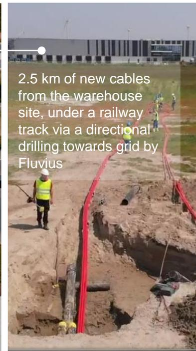
2.5 km of new cables from the warehouse site, under a railway track via a directional drilling towards grid by Fluvius
